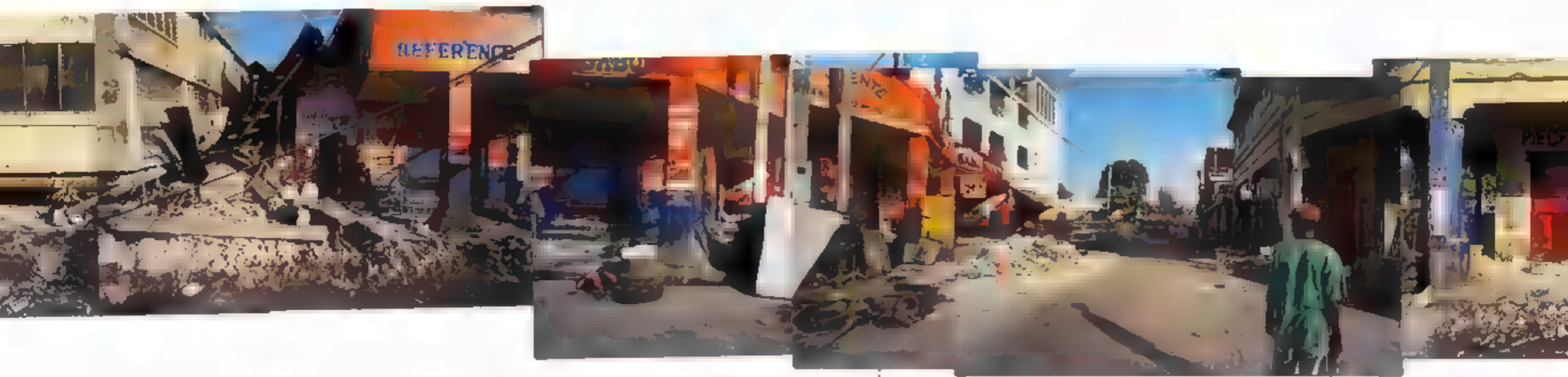
This section of Port-au-Prince's Boulevard Jean-Jacques Dessalines was reduced to rubble.
